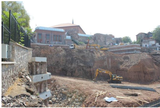
Figure 18. Excavation for the car park, under the mound
