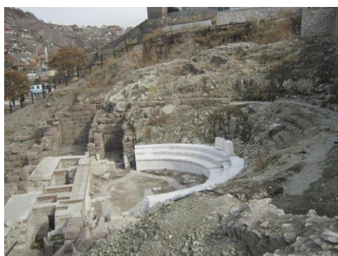
Figure 16. Roman Theater during restoration
