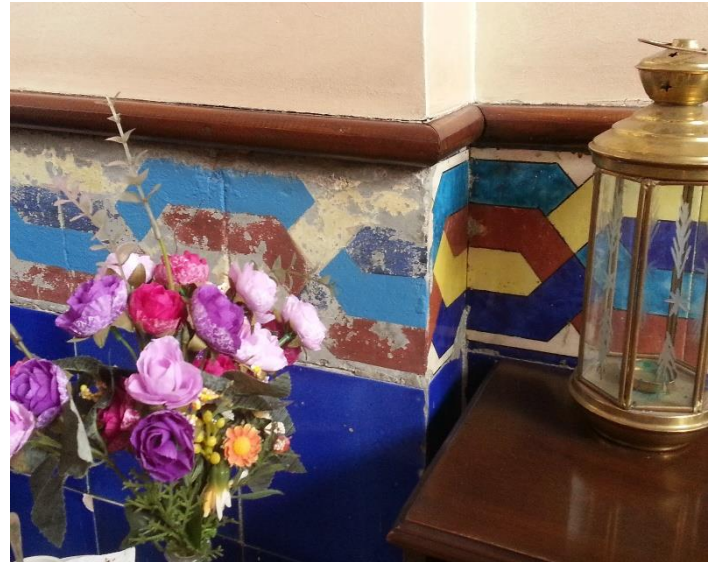
Picture 12, Ankara Gazi Train Station, Inside Wall Maintenance, Özdamar, M., 2015
