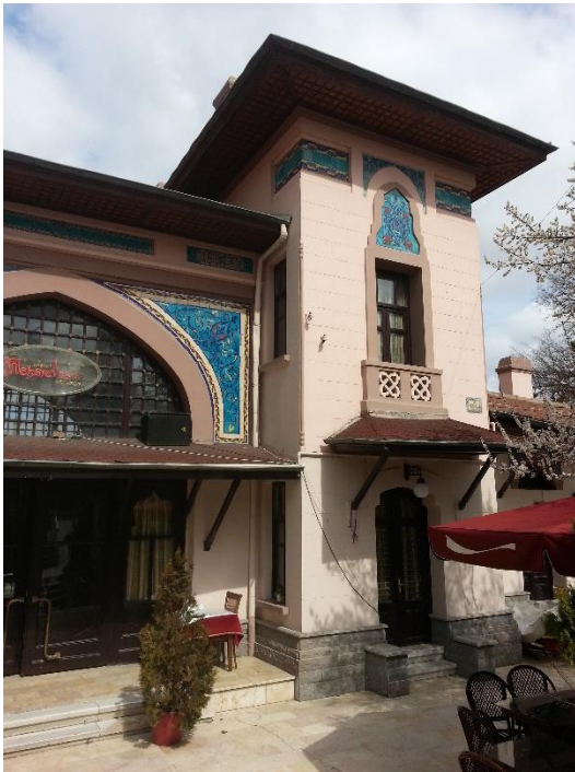
Picture 6, Ankara Gazi Train Station, Front Entrances, Özdamar, M., 2015
