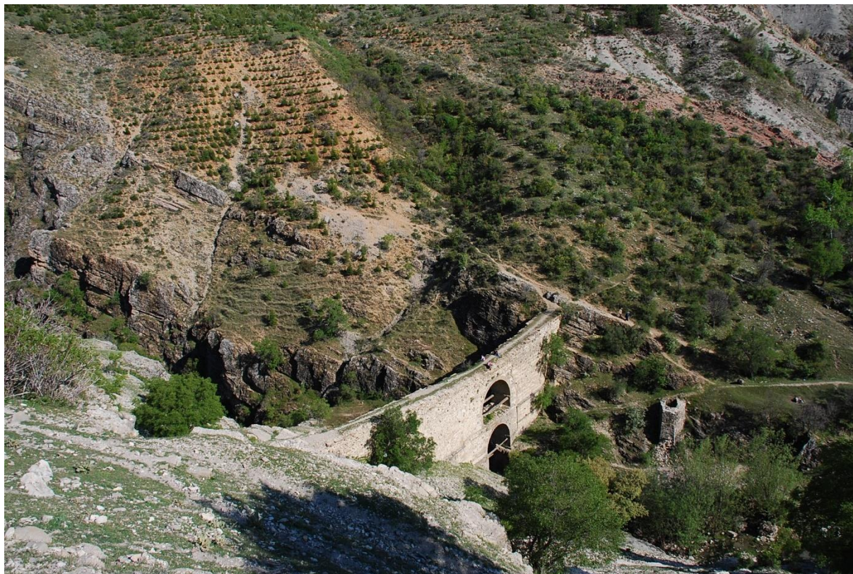
View of Cirimbolu Aqueduct
