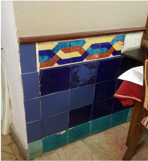
Picture 11, Ankara Gazi Train Station, Inside Wall Maintenance, Özdamar, M., 2015
